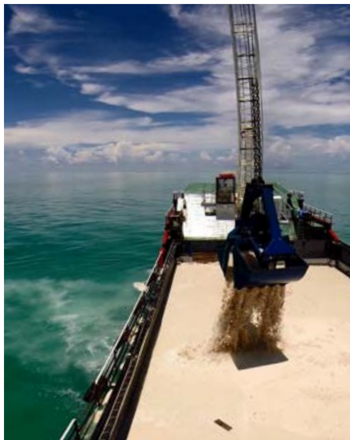
Te Atinimarawa dredging operation (established by the ESAT project) sourcing sustainable aggregate from the Tarawa lagoon.
