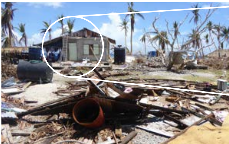
Homes destroyed by Typhoon Maysak in the Federated States of Micronesia. Note: people sheltering in the relatively resilient concrete structure in the background.
