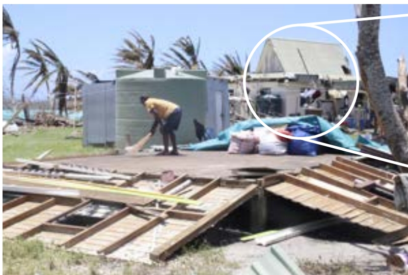
House destroyed by Cyclone Winston in Fiji in 2016. Note the relatively resilient concrete building in the background which was used for refuge during the disaster.
