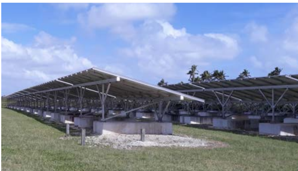
Concrete foundations of a solar farm in Tonga, designed to withstand Cyclone winds.
